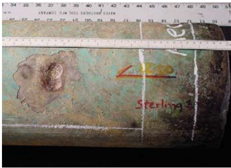
AC Corrosion on FBE Coated Pipeline Leaked 18 months After Installation
