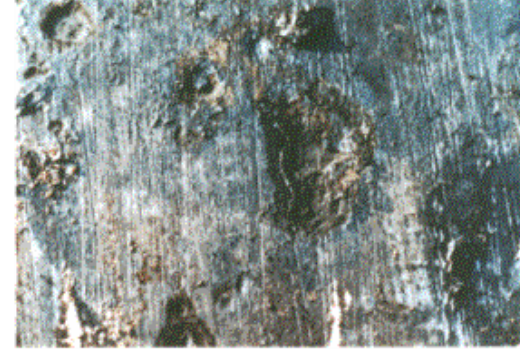
b. Corrosion in pit
