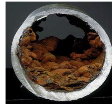
Photo: Extensive tuberculation can discolor and contaminate water as well as result in greatly reduced water flow and pressure.
