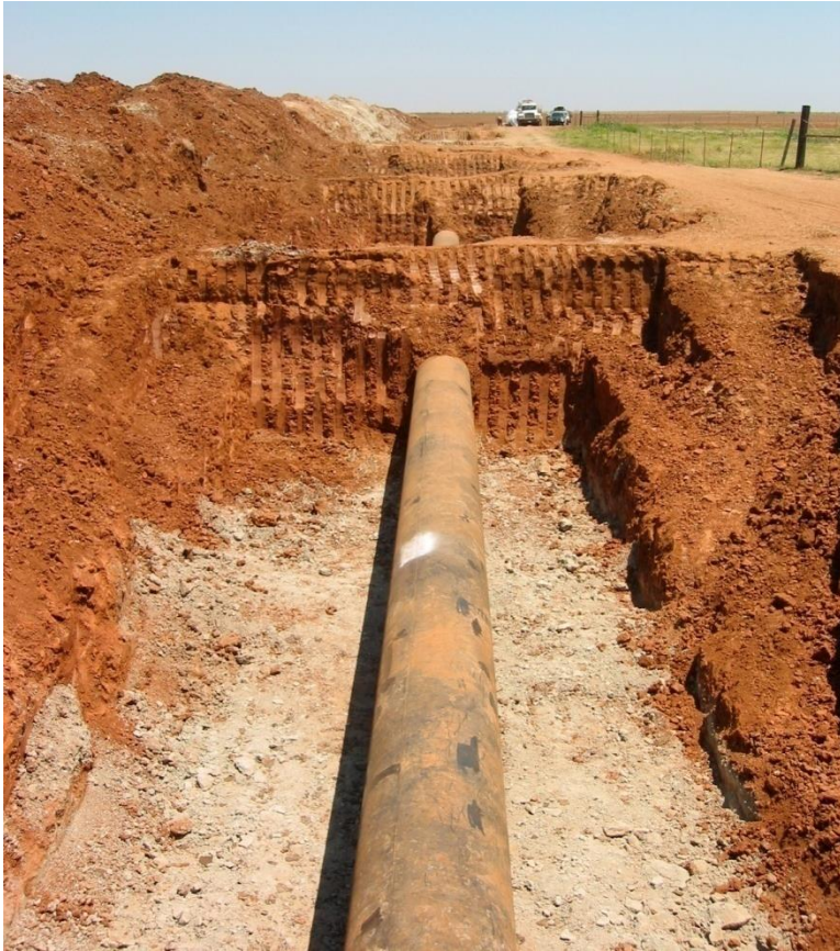
100% Solids Liquid Epoxy Coating - Bell hole rehab - before and after.
