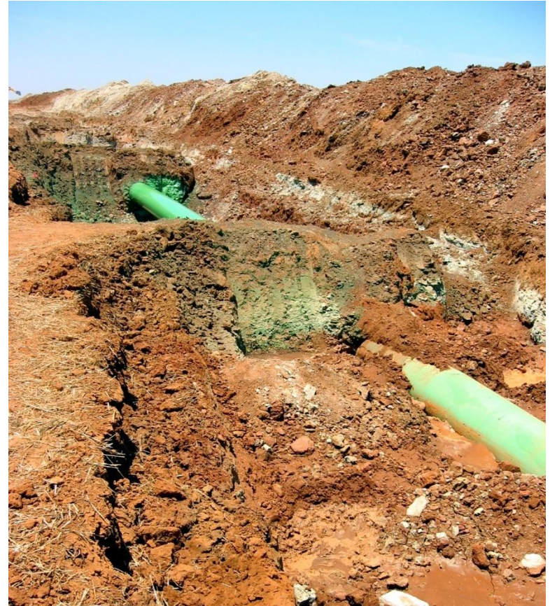
100% Solids Liquid Epoxy Coating - Bell hole rehab - before and after.
