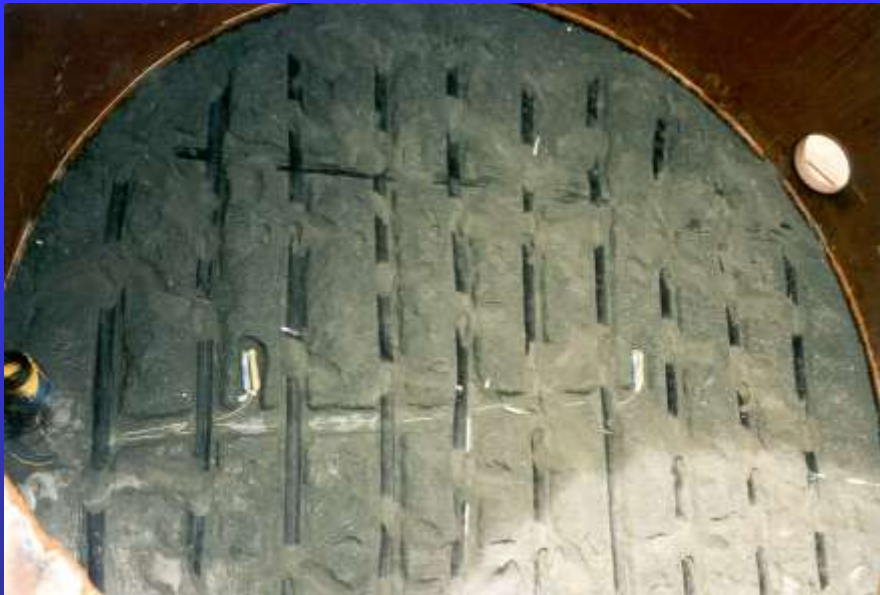
CP Installation on Rebottomed Tank
