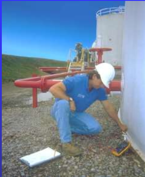
Cathodic Protection Survey (When Tank is Full)
