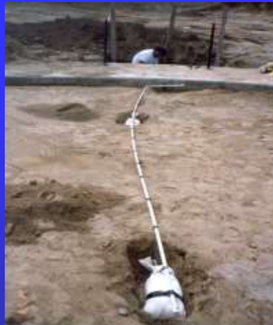
Reference Cell Placement Under Tank Bottom (Note obtain and store native readings)
