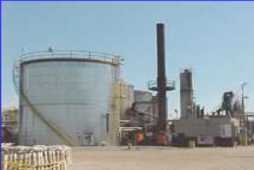
Hot Asphalt Tank Bottoms
