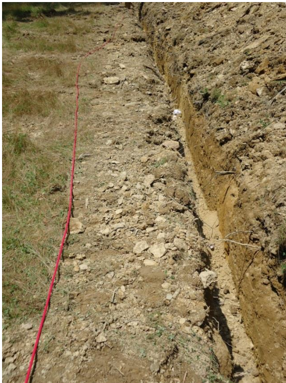
MULTIPLE INSTALLATION OF GALVANIC ANODES
