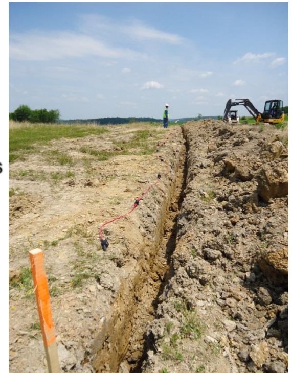
MULTIPLE INSTALLATION OF GALVANIC ANODES
