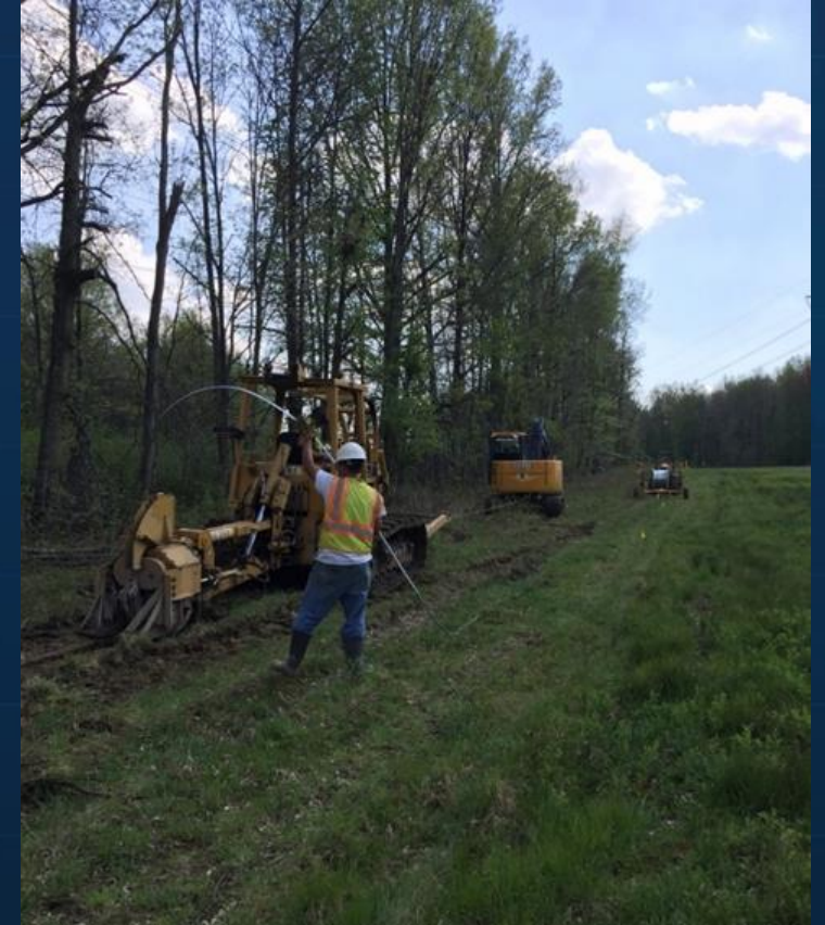
Cable Plow Installing Zinc Ribbon
