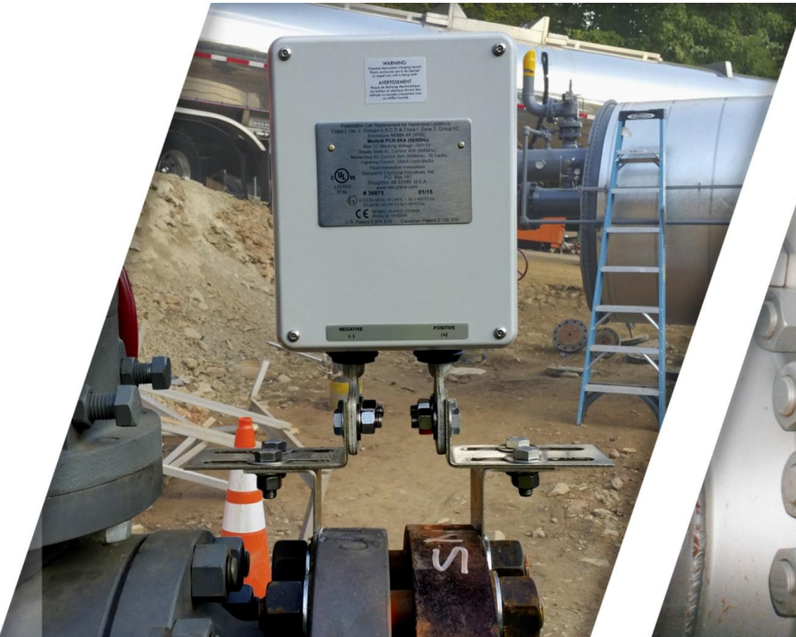
Decoupler on flange bracket
