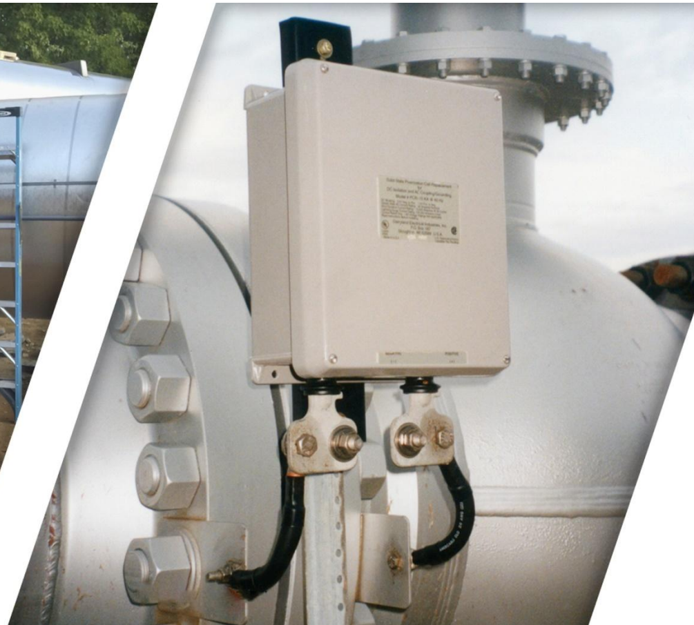
Decoupler on post with flange tabs
