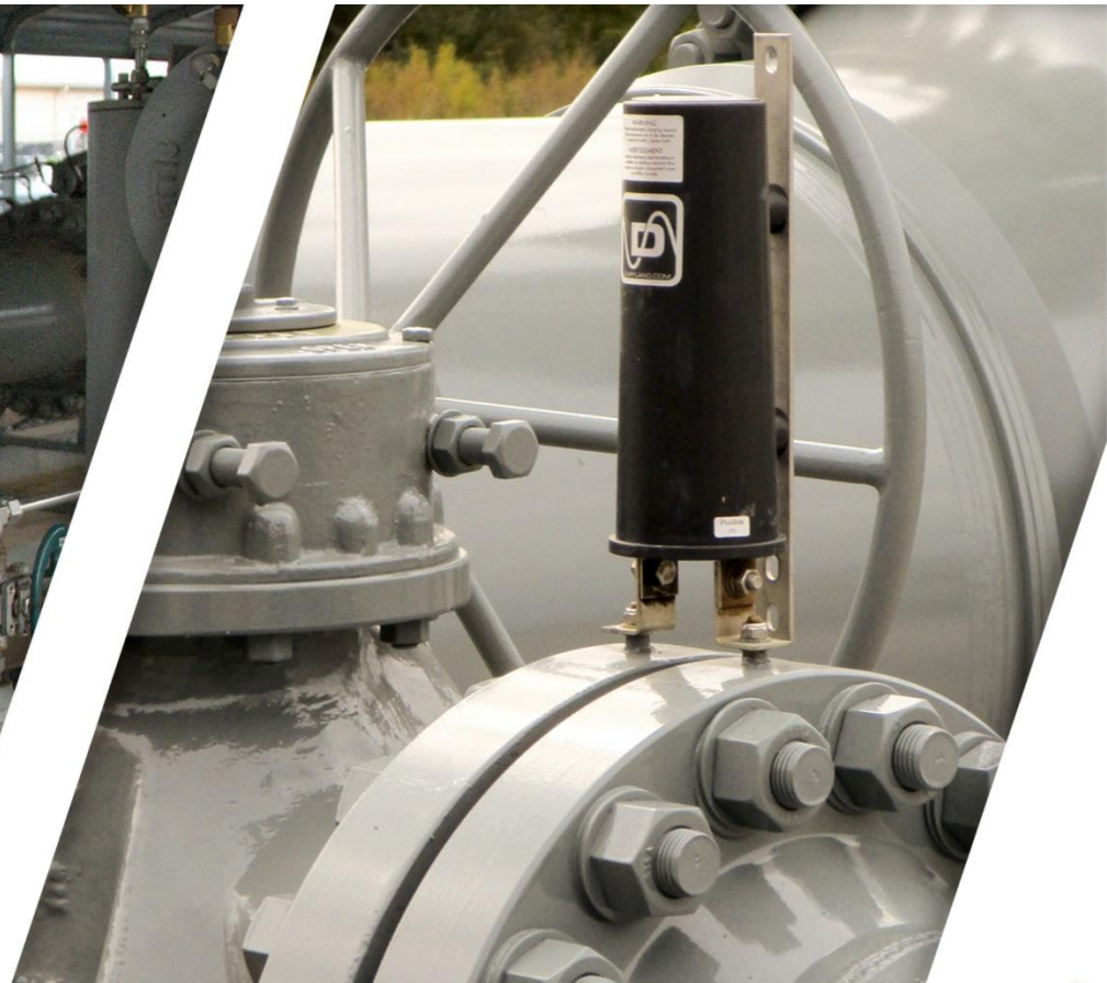
Decoupler on pin-brazed stud bracket
