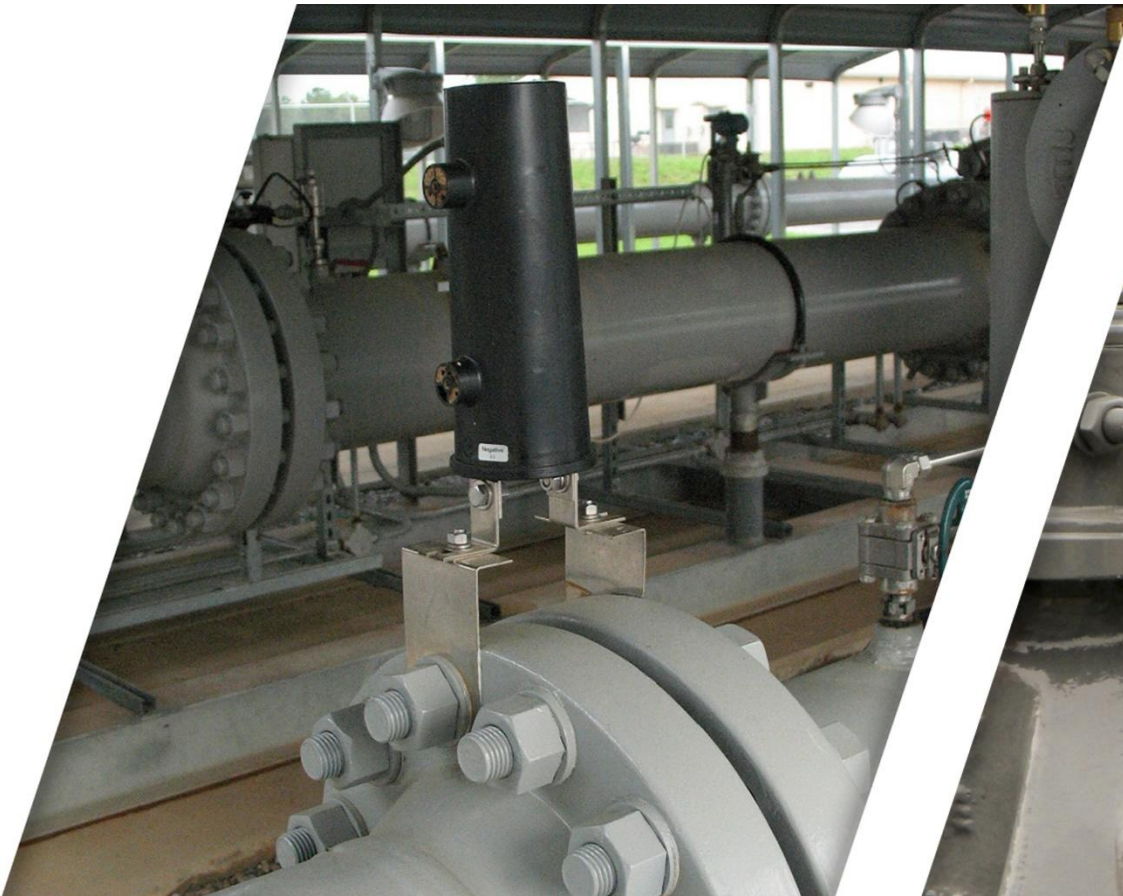
Decoupler on flange bracket
