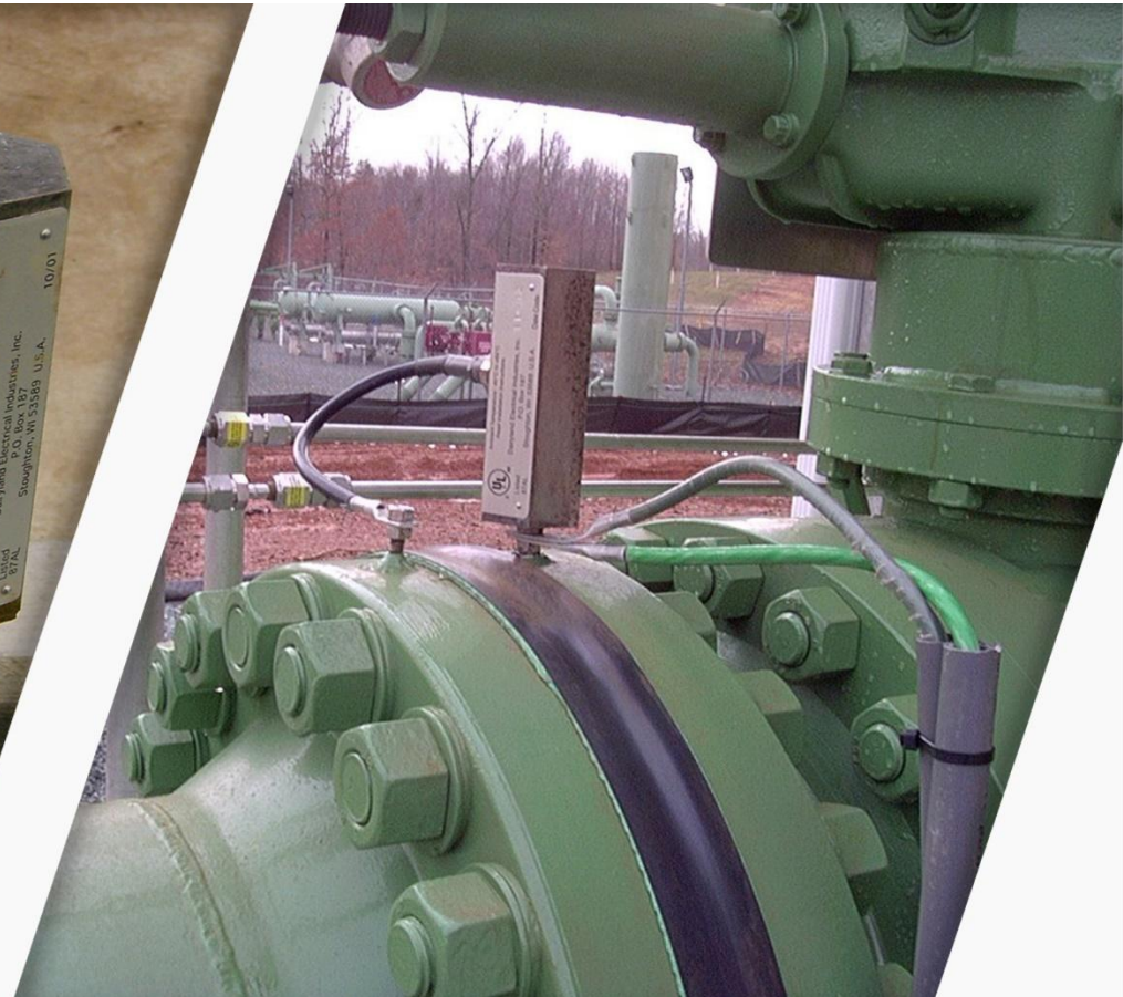
Over-voltage protector on welded/brazed studs
